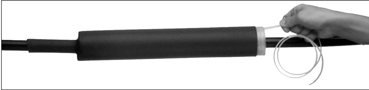
Removing the core
