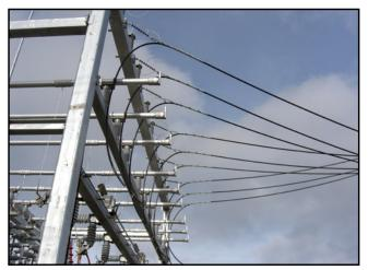
The photo above top shows circuits turning an angle off the last pole outside the substation fence, then running as a slack span (no messenger) into the substation. The photo above bottom shows the phase conductors deadending on the substation bus.
