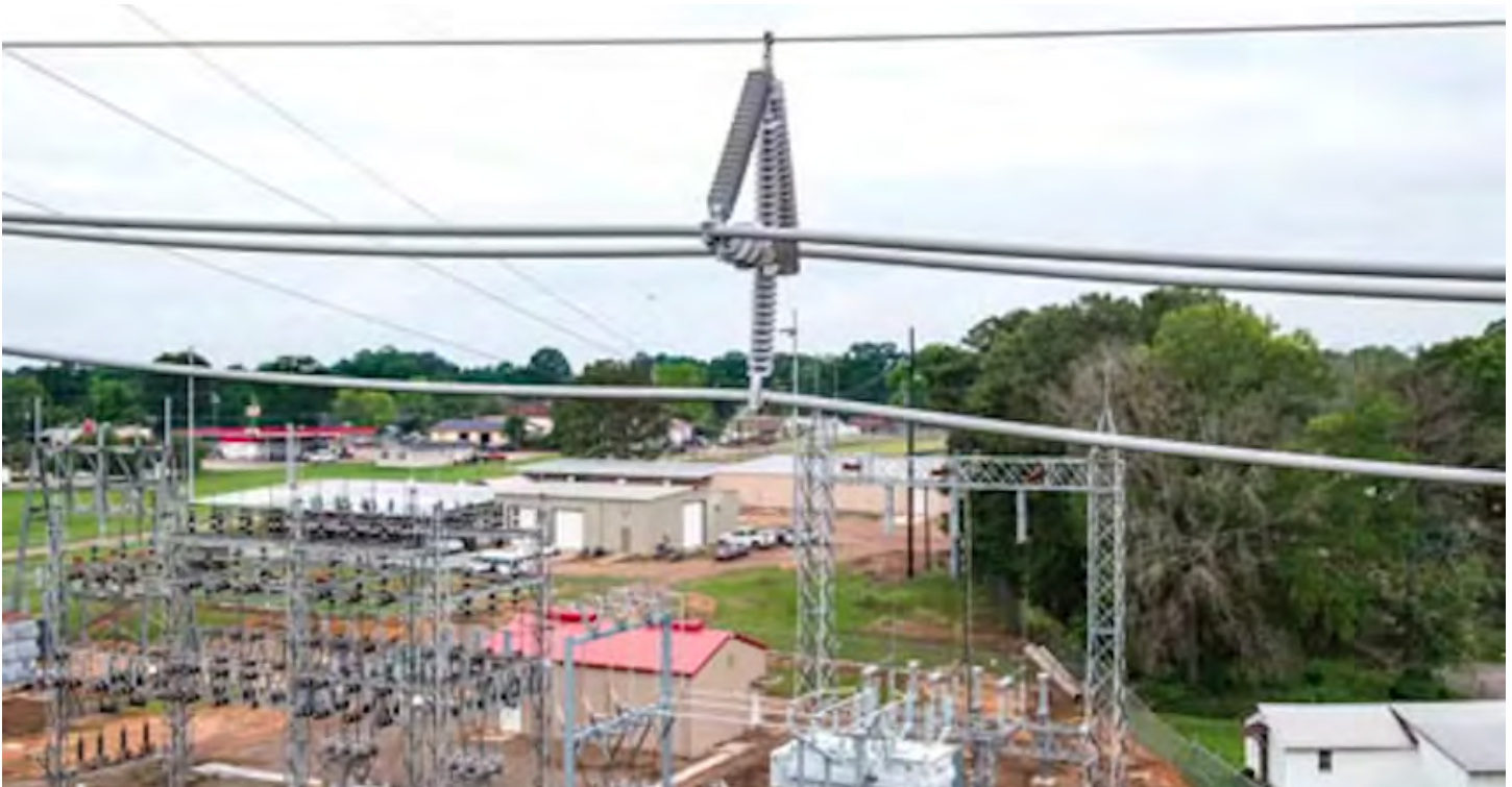
ACS features four individual cables connected using spacer brackets. A heavy-gauge messenger wire that structurally supports the cable system and withstands environmental damage.
