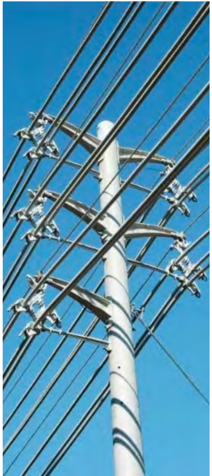
Over- and under-building on poles can increase capacity.
