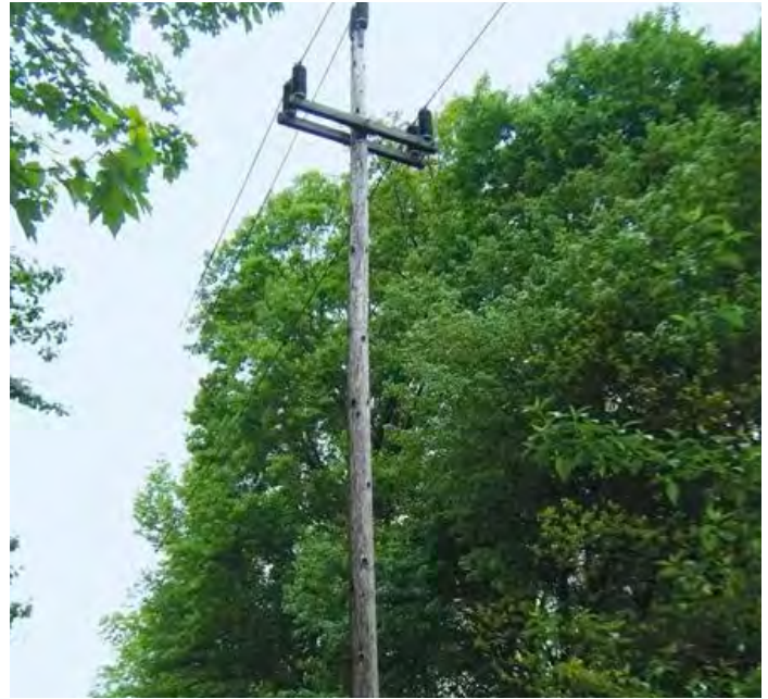
This is typical of the tall trees that are adjacent to the transmission line that experienced all of the outages in 2011.
