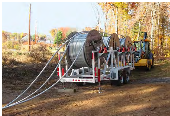
Reels of 69-kV spacer cable ready to be strung.
