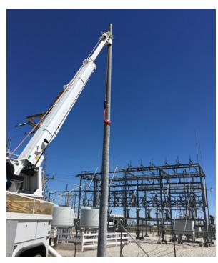
Installation of the riser pole adjacent to the substation.
