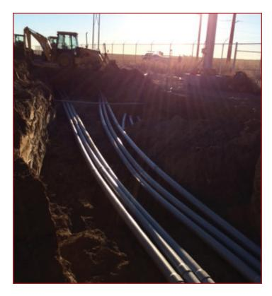
Having completed the underground cable pull, the Kerite and Anderson & Wood crews pulled the cable used for the first circuit that would exit at the South Feeder from ground level to the top of the riser structure inside the substation. The same process was repeated inside the substation for the two circuits that would exit at North Feeders 1 and 2. To complete the three circuits inside the substation, the team installed a total of 18 G&W, 69 kV terminations.
