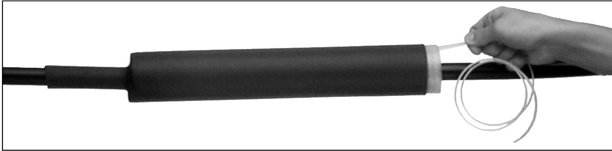
Removing the core
