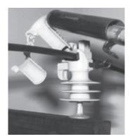
Loosen the bolt and slide the VTST-1 away from the insulator, either by hand or with a hot stick, until the two halves of the tool separate
