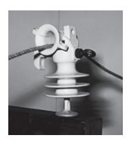
Install the Vise Top Insulator. Clamp the VTST-1 in the jaw and pull your rope in (Hint: have the large flare of the VTST-1 facing the cable reels)
