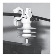
String and sag the conductor directly on the insulator. Dead ends can be made up and the circuit can be energized (remember: you are in an insulator)
