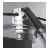
Clamp the conductor in the Vise Top jaw by tightening the torque bolts, BOTTOM BOLT FIRST — ALWAYS, until the rings break away. This can be done by hand or hot stick
