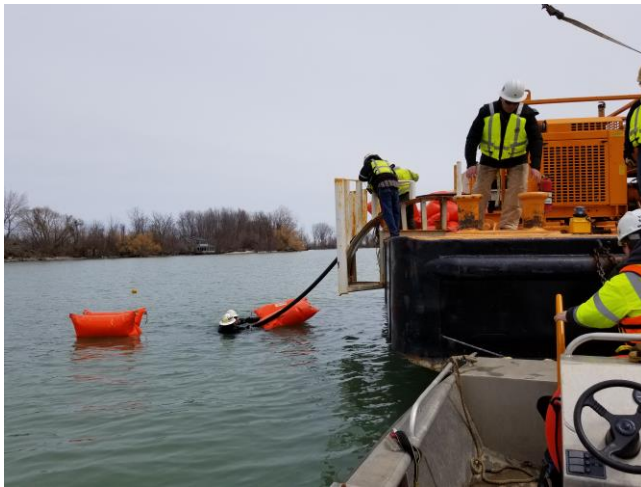
Cable laid directly on lake bottom
