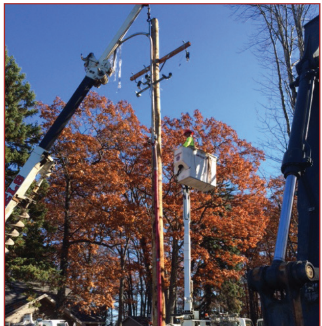
Setting the new riser structure on the feed side
