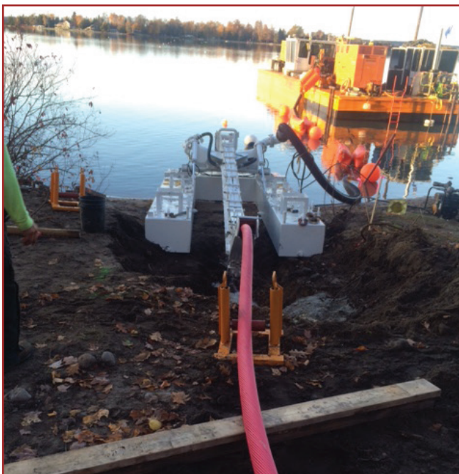
Jet Plow on land side of cable run
