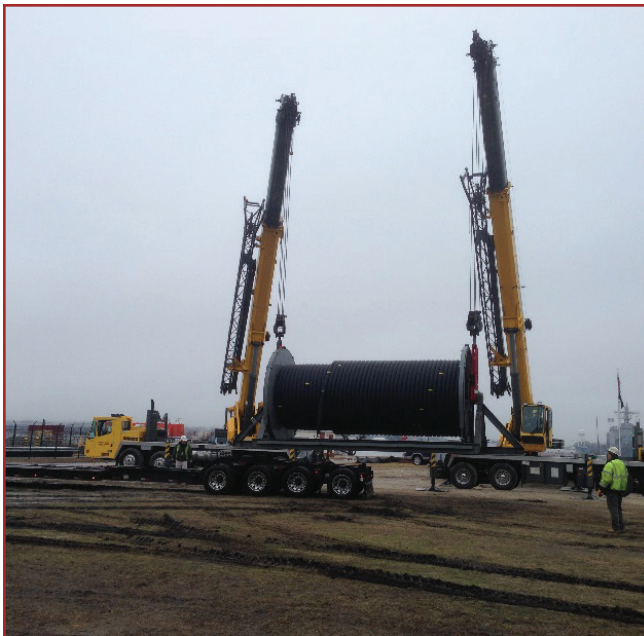
50 ton cable reels being offloaded in Virginia Beach
