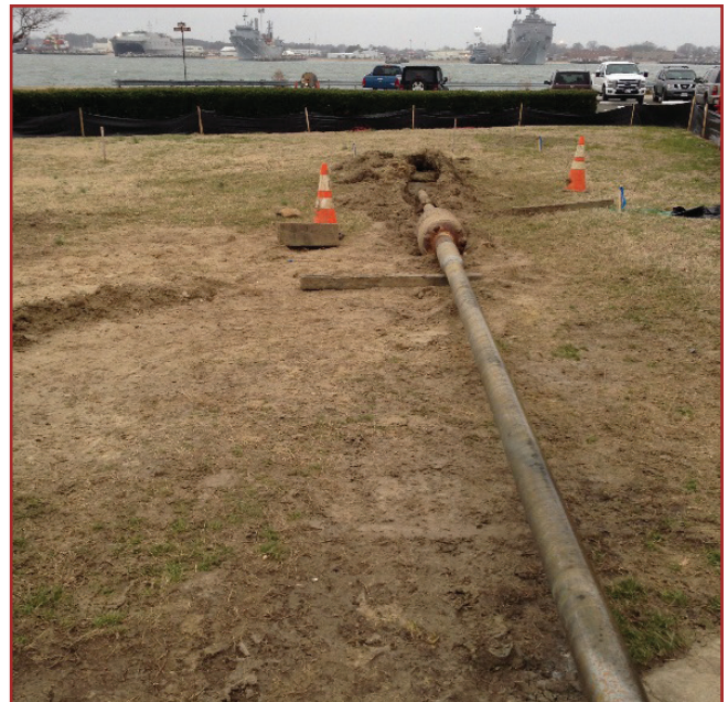
Directional drill across Little Creek at the Amphibious Naval Base
