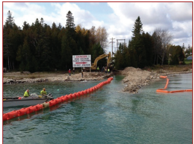
Floating the cable to shore to be terminated.
