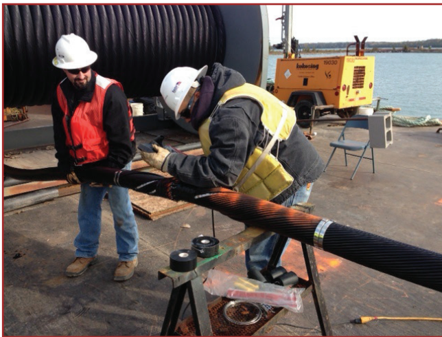
KCS Technicians cutting the armor wires back on the cable.
