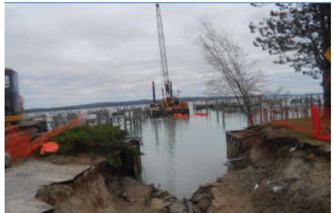
Subsea cable being laid off of barge.
