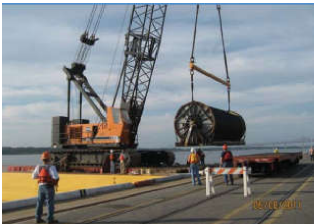
Loading cable reel onto barge.
