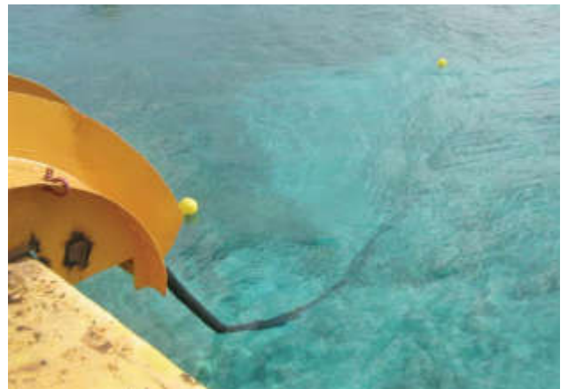
Subsea cable being laid off of barge.
