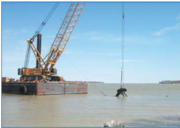
Barge excavating trench in Lake Erie.
