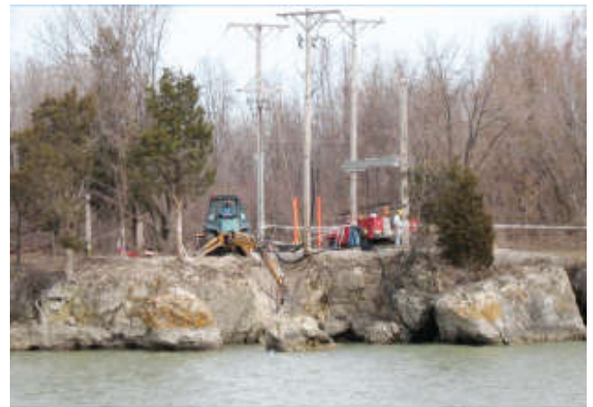
Building concrete bulk head, Middle Bass Island.
