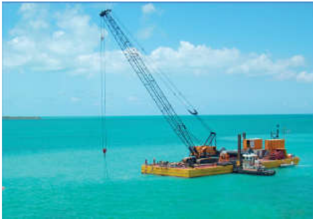
Barge used in cable installation.
