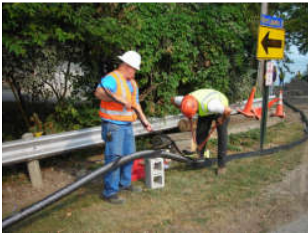
KCS Technicians removing armor wires from the new subsea cable.
