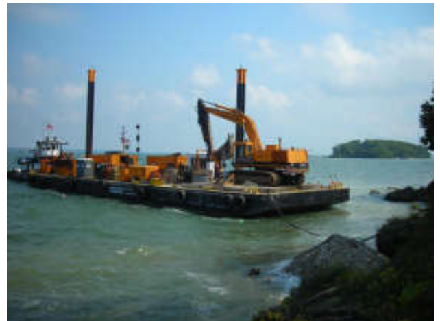
Durocher Marine prepping the barge for installation.
