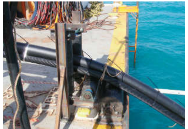
Cable and Water Line Installation.
