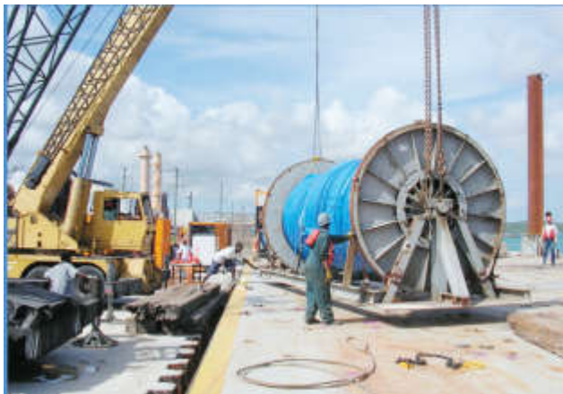
Loading Cable Reel on Barge.
