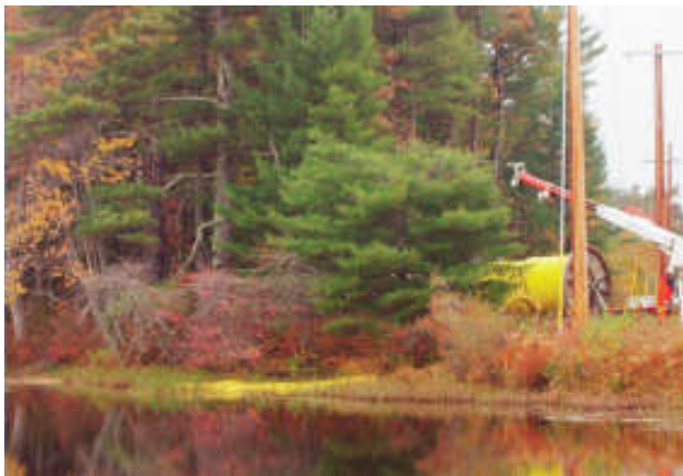
Cable Lay Operation
