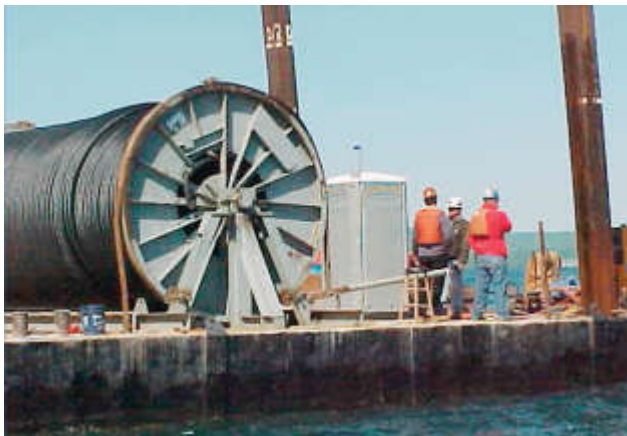
Cable Lay Barge.
