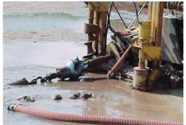
Horizontal Directional Drill.
