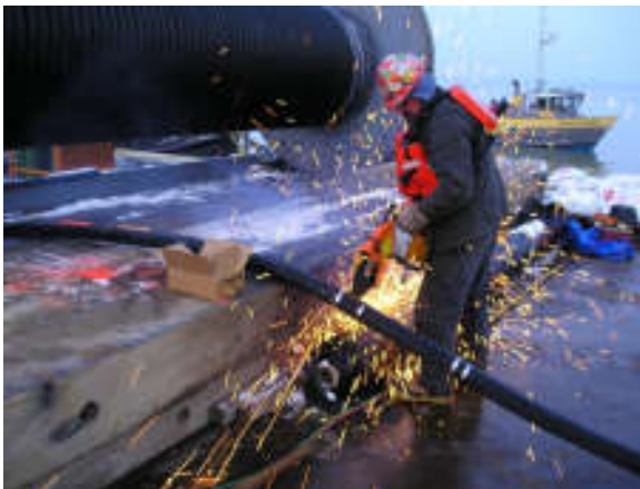
Cutting the cable to float to land.
