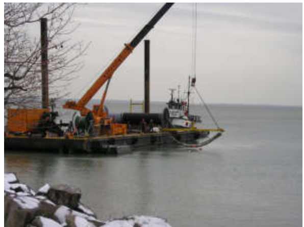
Installing articulating concrete block mats for cable protection.
