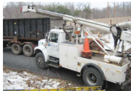
Removal of Self Contained Fluid Filled Cable.
