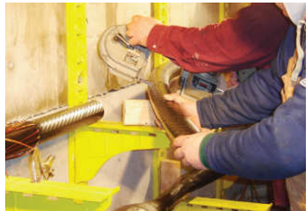
Cable Splice Preparation.
