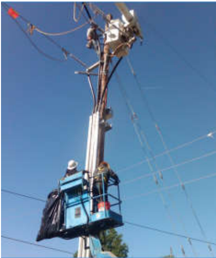
Crews working on pole outside of substation.
