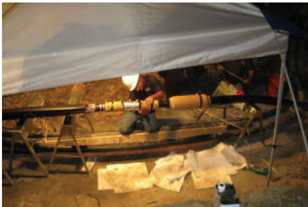
Installation of splice.
