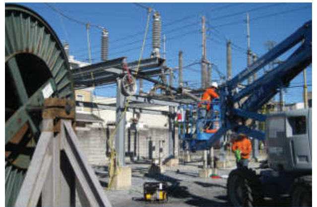
Pulling cable in substation.
