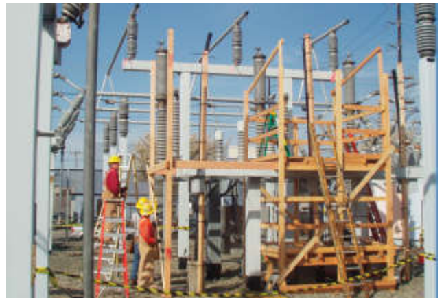
Platform constructed to facilitate installation of termination.
