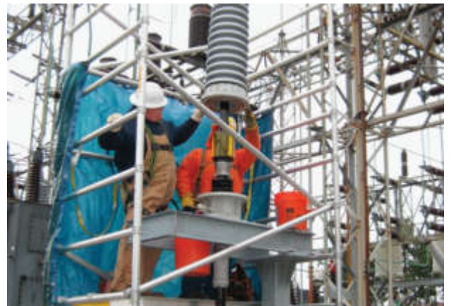
Removal of old termination.
