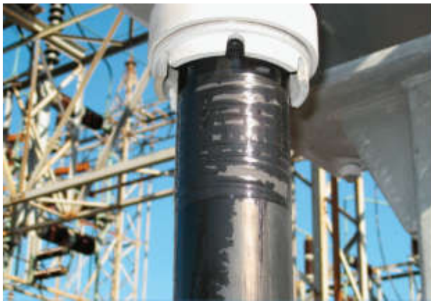
Termination leaking.
