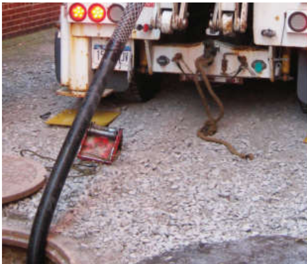
Removal of cut cable.
