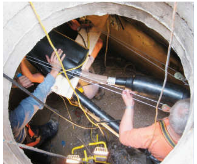
Installation of Elastimold premolded splice.
