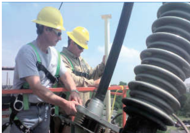
KCS technician building HV termination.
