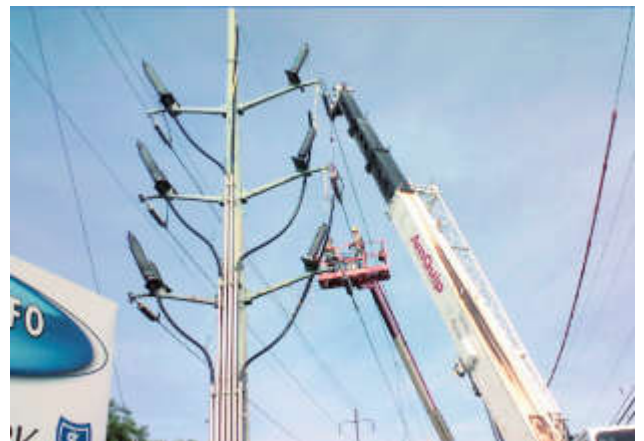
Completed HV terminations.
