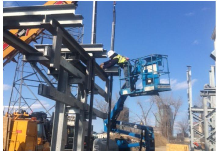
This time around, Eversource and the teams had to install a single circuit of the 1000kcmil Cu 115kV underground cable to officially complete the project. In just a short six-day period, the crews installed three 150 foot lengths of power cable, along with another six G&W PAT 140 terminations atop the new termination riser structures. Kerite Cable Services and CCCC took care of the shield grounding and performed the final acceptance testing of the new circuit before it was energized.
