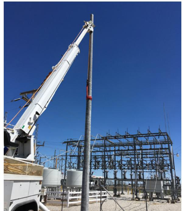
Installation of the riser pole adjacent to the substation.
