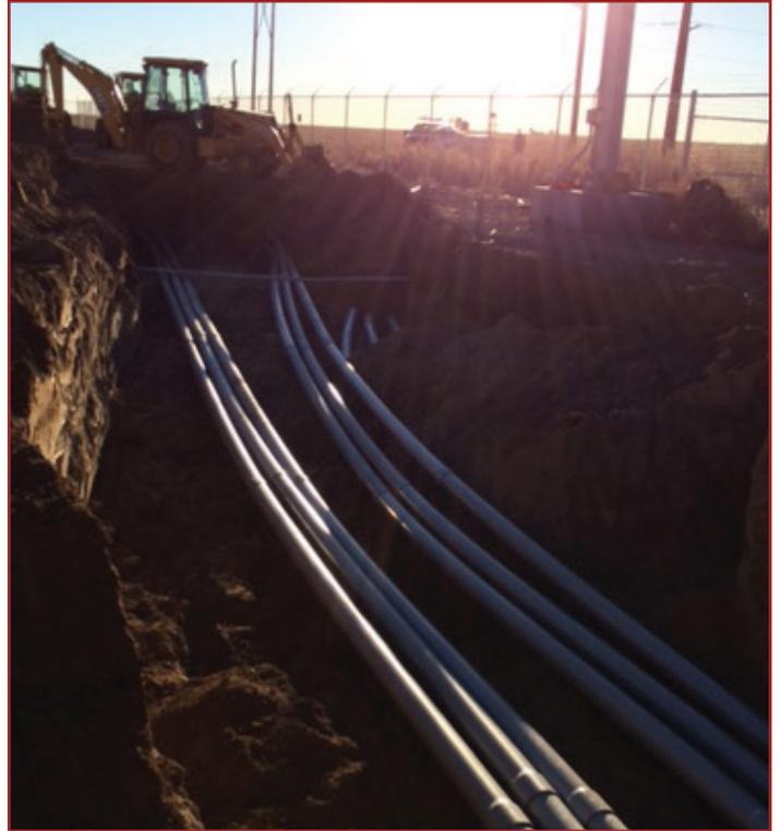
Having completed the underground cable pull, the Kerite and Anderson & Wood crews pulled the cable used for the first circuit that would exit at the South Feeder from ground level to the top of the riser structure inside the substation. The same process was repeated inside the substation for the two circuits that would exit at North Feeders 1 and 2. To complete the three circuits inside the substation, the team installed a total of 18 G&W, 69 kV terminations.
