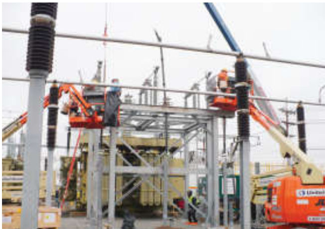
KCS technicians work in tandem to meet the required time constraints.
