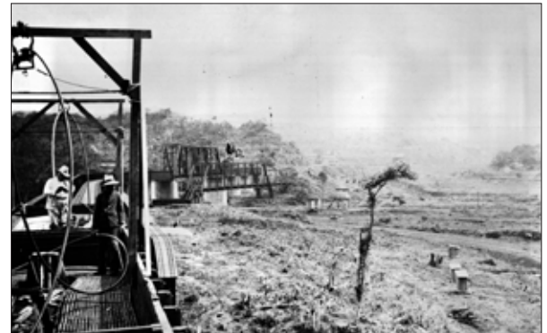
Panama Canal cable installation, 1908
