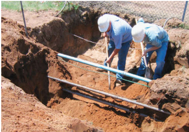
Hand Excavation Near Existing Utilities
