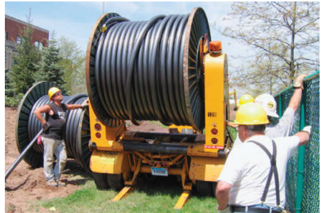
Preparing To Pay Off Cable Into Trench
