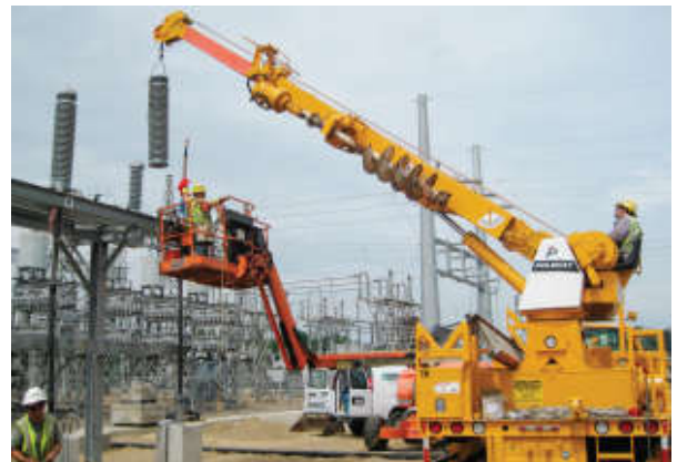
Installing porcelain termination
