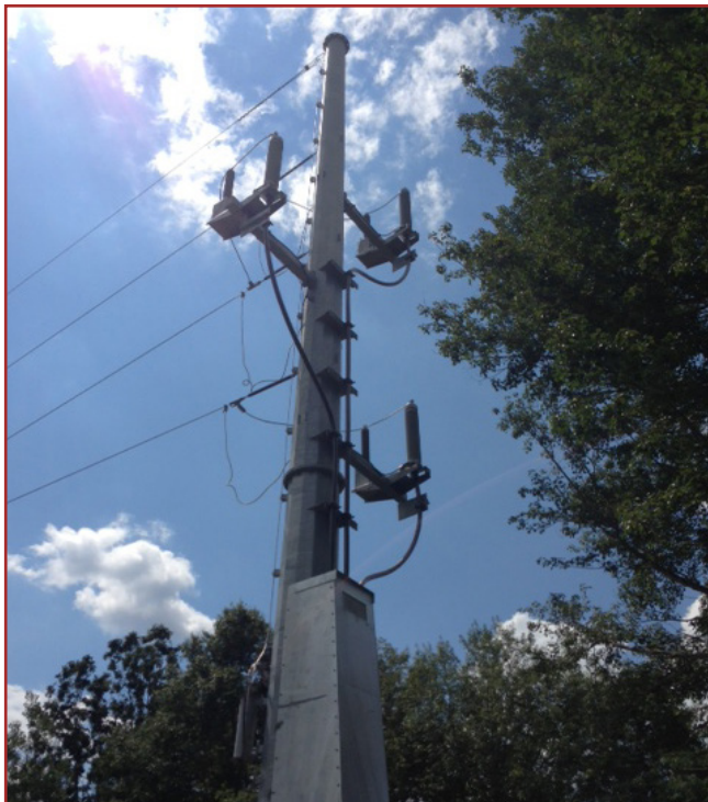
Completion of G&W PAT 140 Terminations on 78' transition pole.
