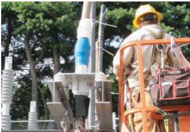
Installation of G&W Stress Cone.
