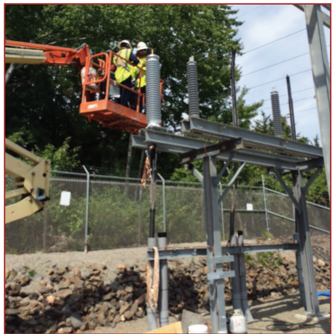
KCS technicians assembling a G&W PAT 140 termination
