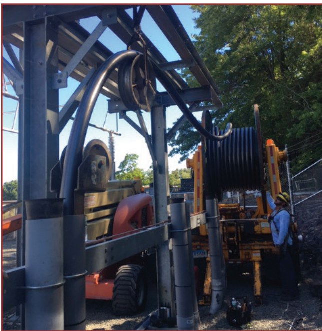
Pulling cable into duct bank
