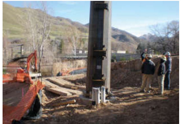
Pole ready for cable installation.
