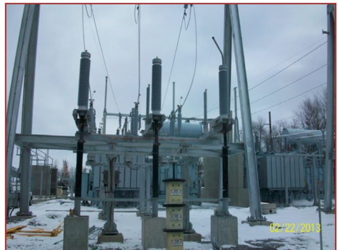
Final system acceptance testing 240kV DC Hi-POT.
