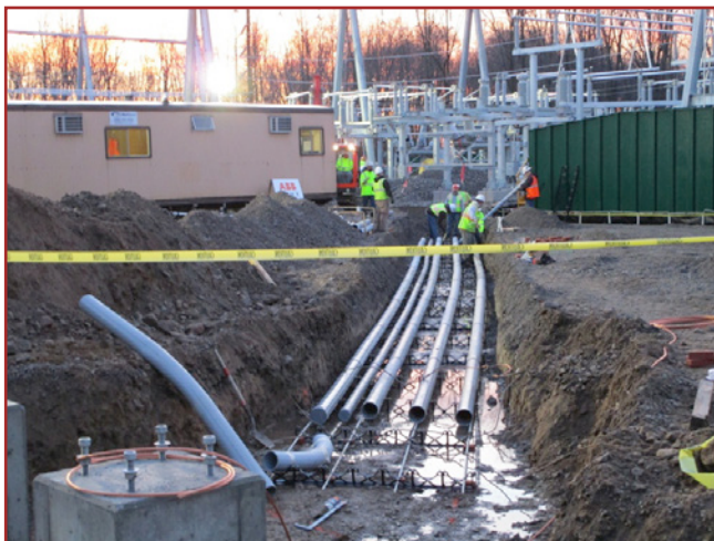
Construction of owner installed concrete encased duct bank.
