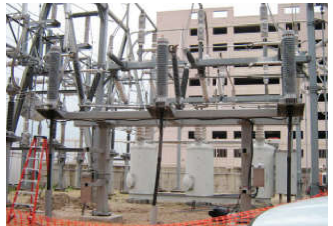
Completed terminations within substation.
