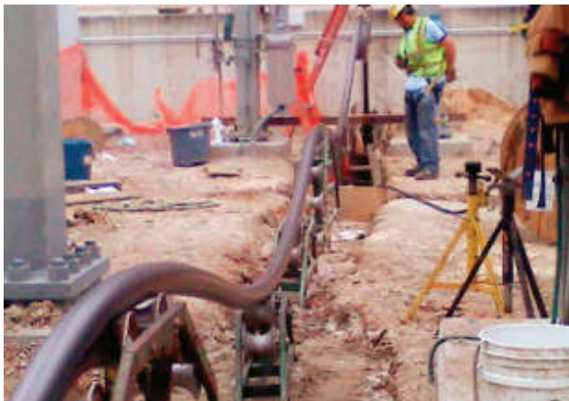
Cable pulling across substation due to space constraints.
