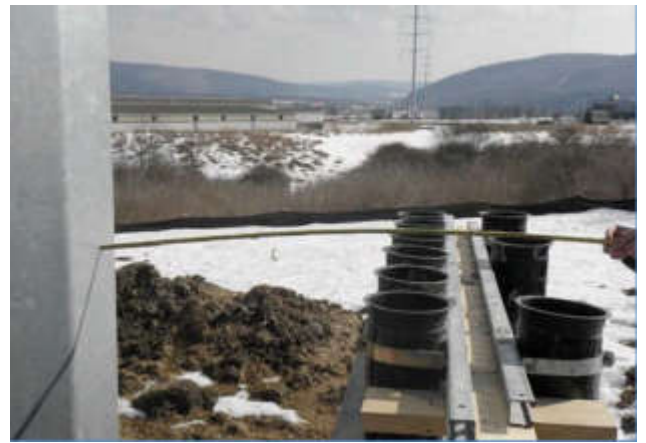
Double circuit duct bank.
