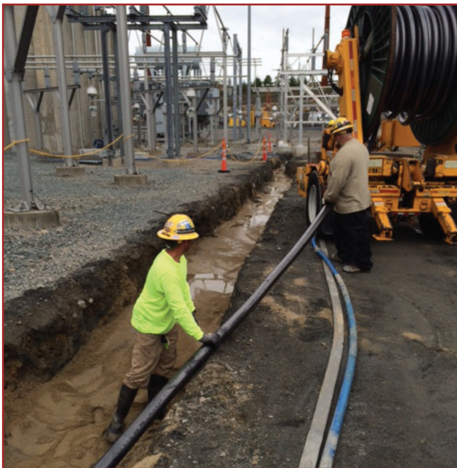
Laying cable in trench. Cable was direct buried.
