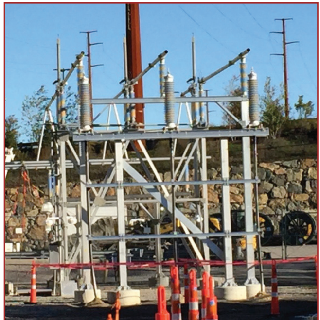
Completed 3M TP-123 terminations.
