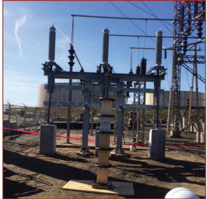
DC Hi-Pot testing @ 226 kV
