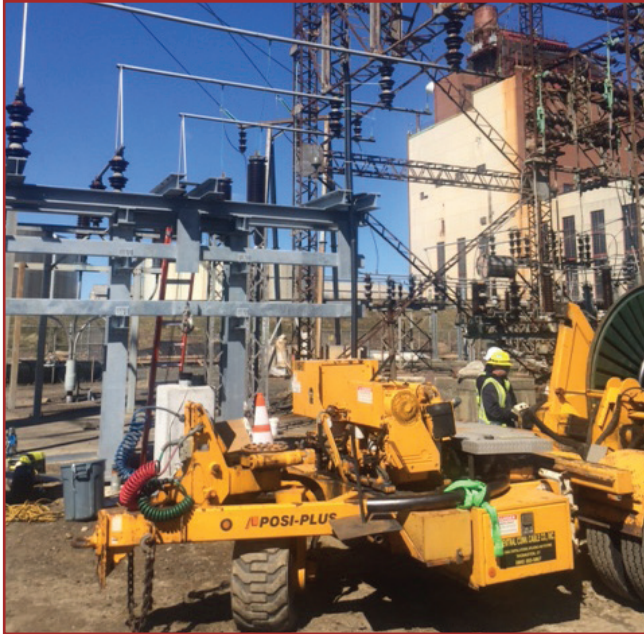
Pulling the cable up the riser structure
