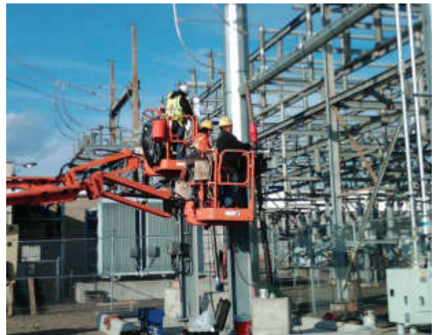
Two crews installing high voltage termination.
