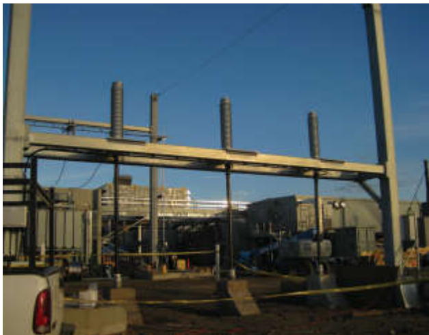
Completed high voltage termination.
