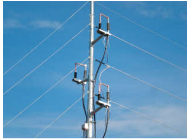
Completed terminations with link box and bus work.
