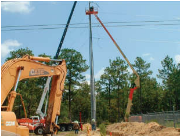
Pulling cable up 90ft pole.
