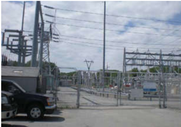
Kent County site, working with close clearance to overhead lines.
