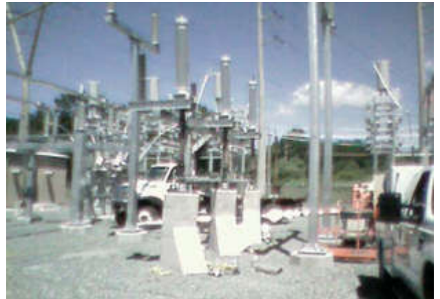
Completed structure with polymer terminations.
