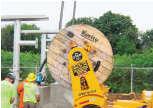
Cable pulling with Central Connecticut Cable Company.
