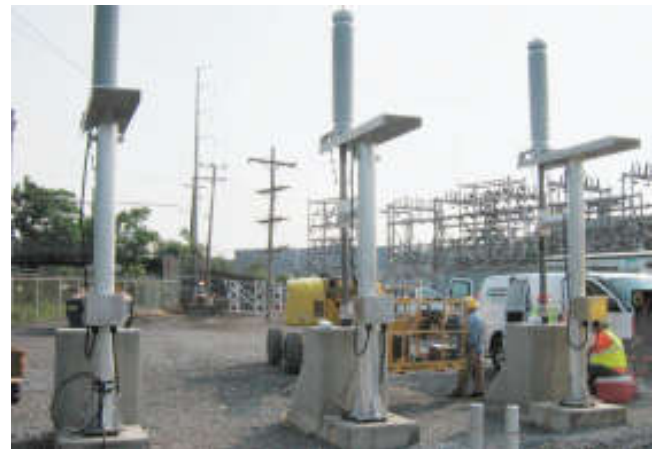
Finished 115 kV terminations. Job completed in 8 days.
