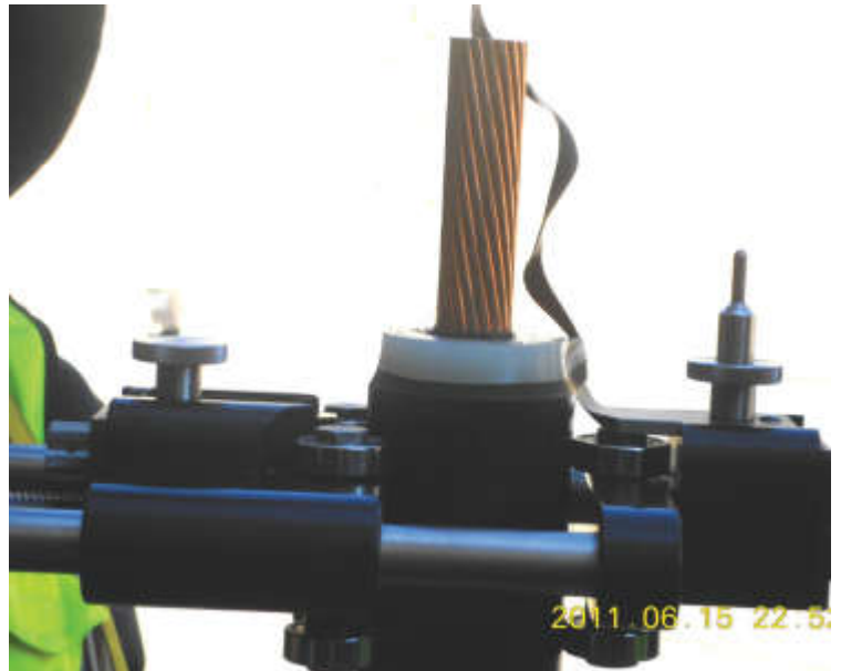
Using specially tools to remove insulation shield.
