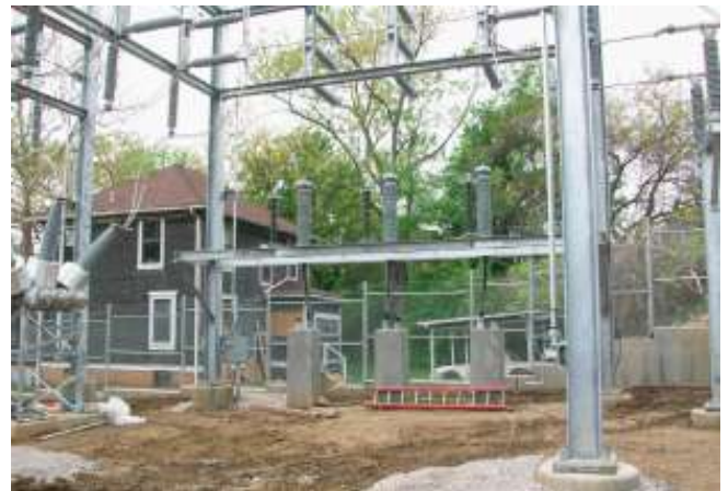
Completed G&W terminations.
